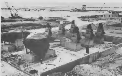
EARLY STAGES of construction of the ACI fertilizer works dot the area west of the Antilles ammonia plant. Prominent among the buildings is the compressor house, above, for the urea plant. In the far background is the lagoon and the workings involved in pier and dockside construction.
